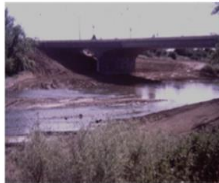
Pedrick Rd. Bridge, 1974, University mines gravel from creek and bridge construction
