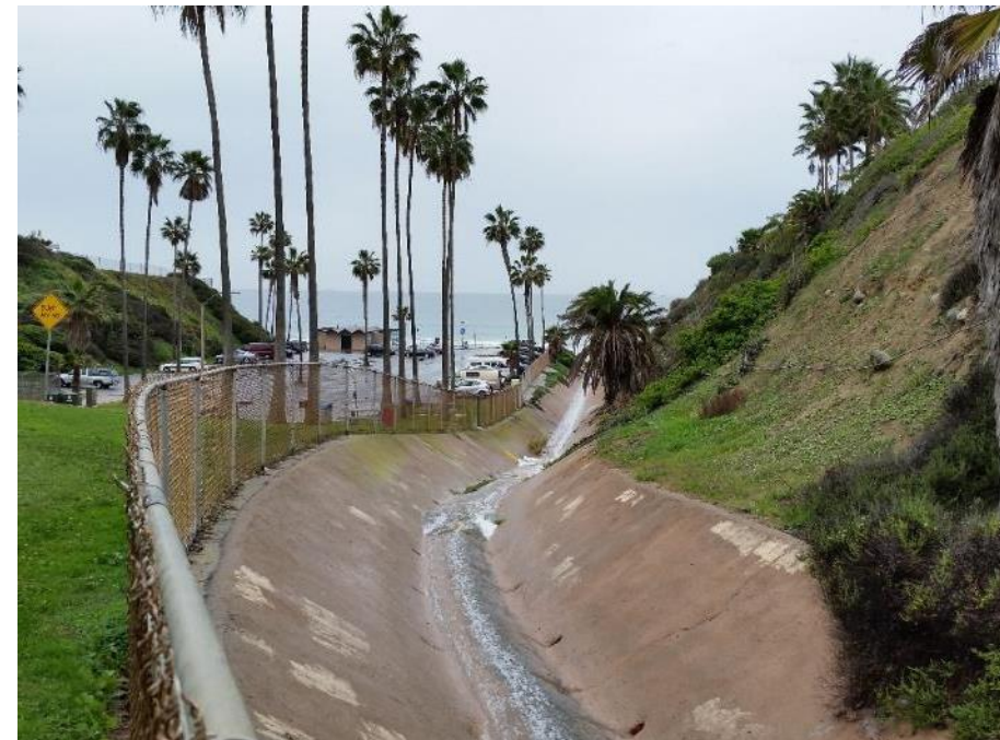
Urban stormwater at Tourmaline Beach in San Diego, CA
