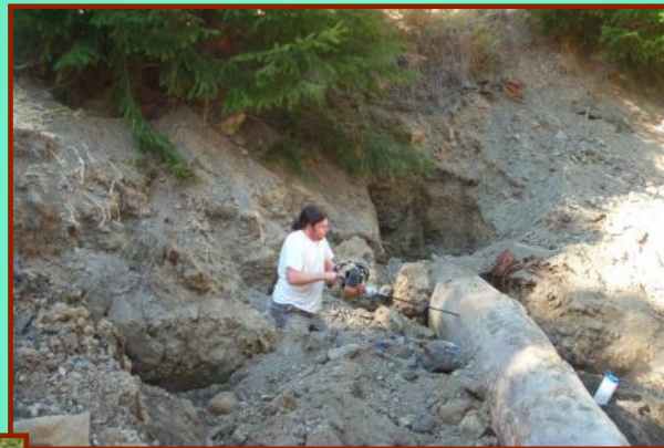
In-stream Structure Implementation
