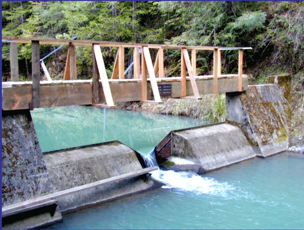
North Fork weir under varying flow conditions
